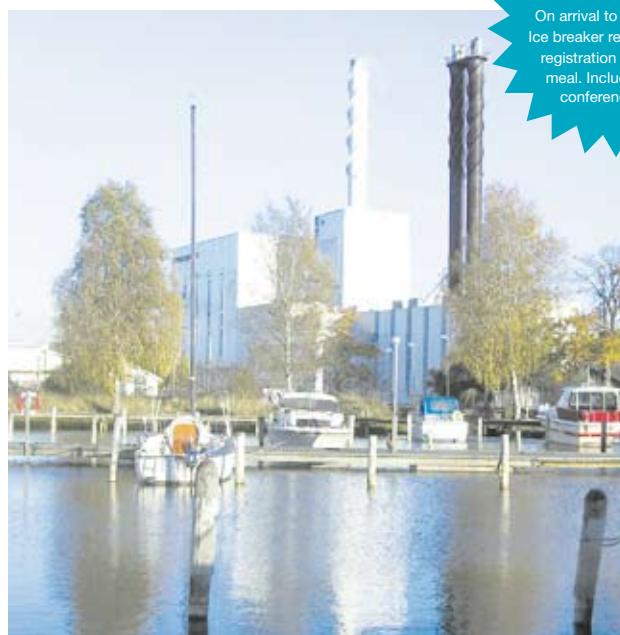
Biomass CHP plant delivering 50 % electricity and 100 % heat to inhabitants in Enköping.
