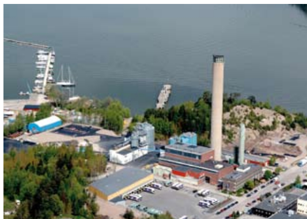
Biomass fuelled combined heat and power (CHP) plant, Fittjaverket.
